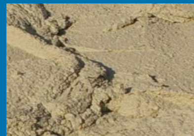
80 pcf cellular concrete during placing
